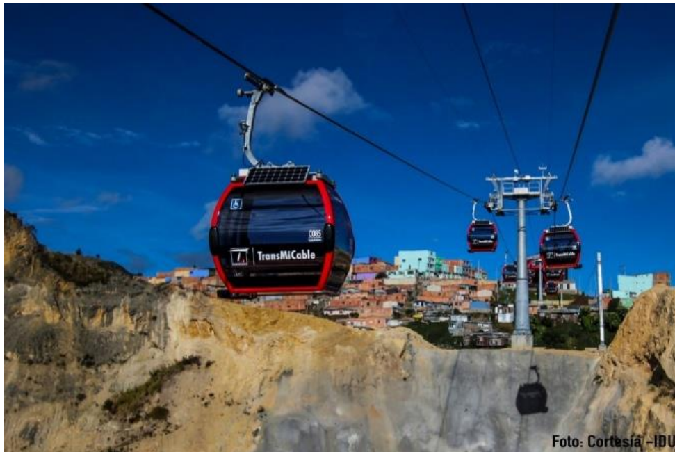
Figura 3 TransMicable Portal Tunal
